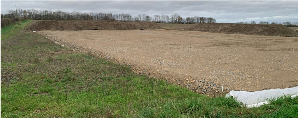
Photo 14: Newly laid Construction Compound (Elsham–Lincoln Pipeline)
