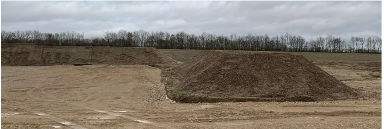
Photo 16: Topsoil Storage Example (Elsham – Lincoln Pipeline)
