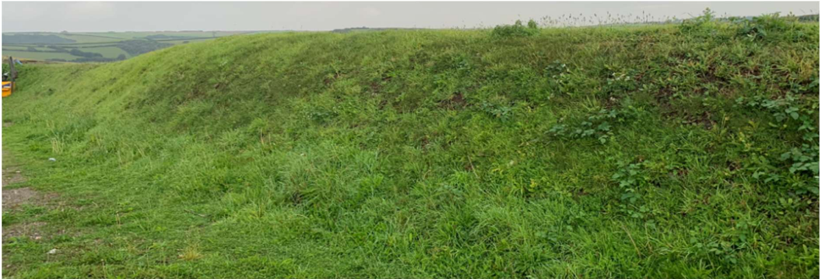
Photo 17: Grass-seeded Soil Storage
