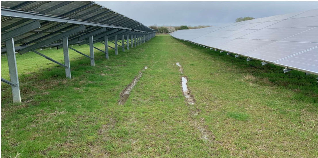
Photo 29 28 : Ruts Caused by Vehicles
